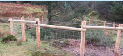
A fenced off mine shaft
