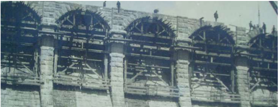
Doing the final touches to the dam
