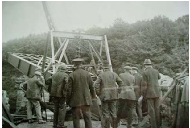
The pillars of the suspension bridge being erected
