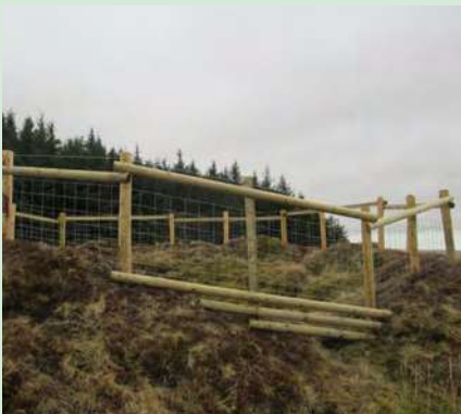
The new wooden gate and fence
