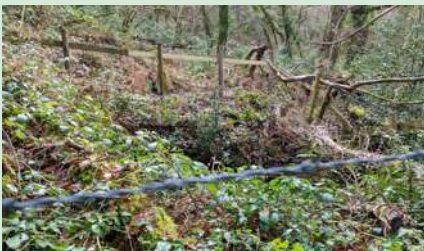
Part of the new fencing
