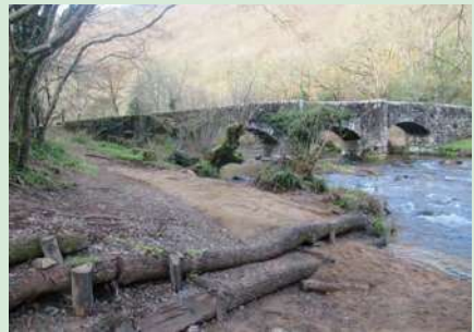
Part of the river bank repairs
