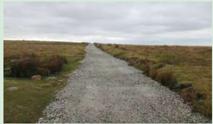
Part of the new surface
