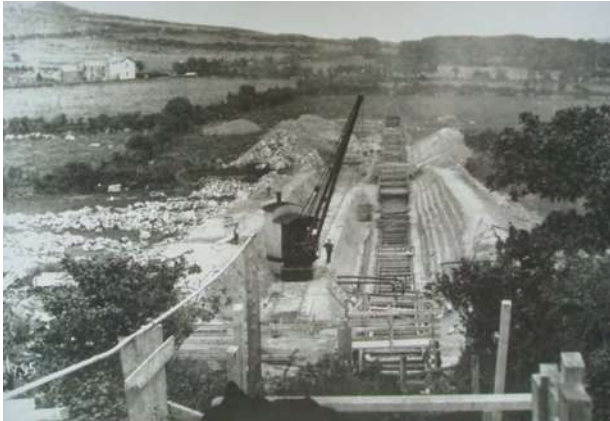
Sheepstor Dam being built
