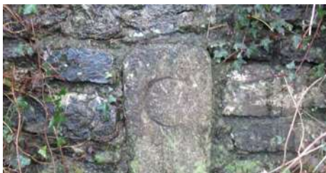
The cleared C stone at Dart Bridge
