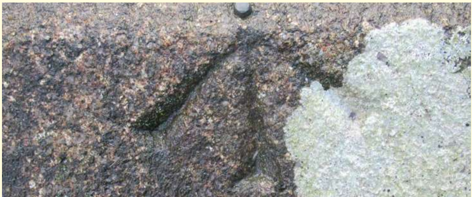
The benchmark on the parapet
